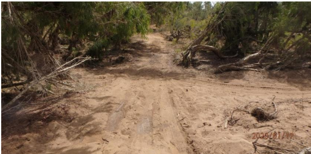
Figure 3-10 Existing crossing to Big Bend
