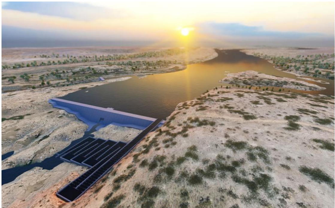
Figure 3-2 Digital visualisation from downstream of the weir looking upstream
