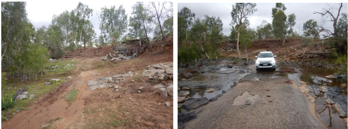
Figure 3-13 Typical condition of existing access track (left) and Lolworth Creek crossing (right)
