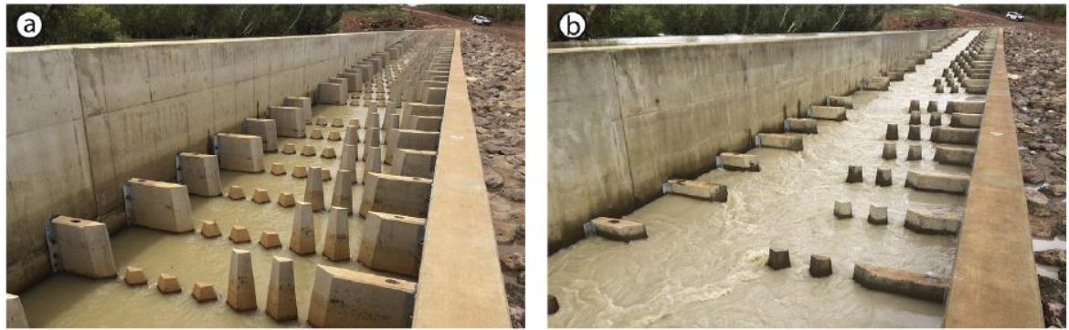
Figure 3-5 Glenore fishway at low (a) and high flows with low turbulence resting areas (b) (extract from Stuart and Marsden 2019)
