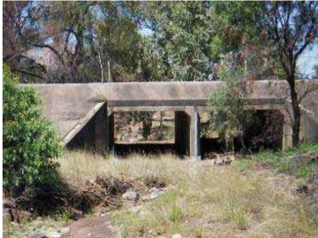
Horse Creek crossing culverts, looking downstream
