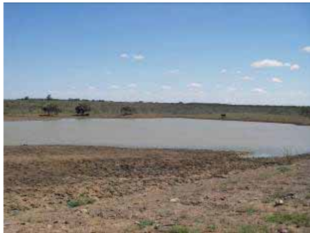
Dam looking upstream
