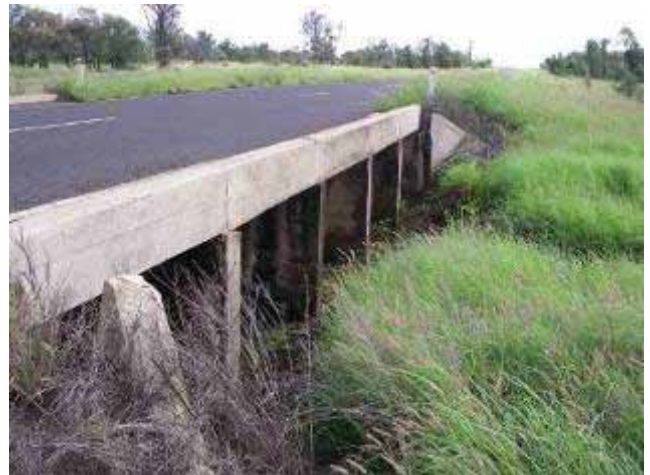
Five box culverts
