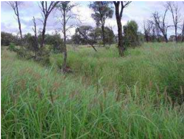
Culvert crossing and creek
