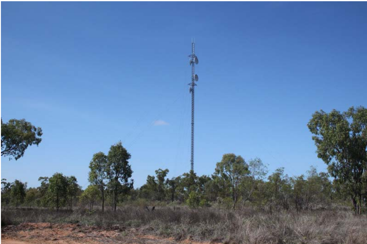
Plate 3-1: Telecommunication tower contained on Lot 1 BL55
