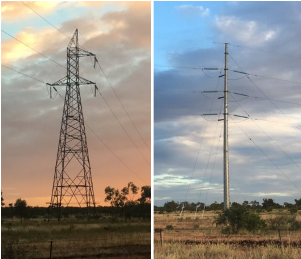
Plate 18-2 Typical 220 kV single circuit lattice transmission tower (left) and 220 kV single circuit monopole (right)
