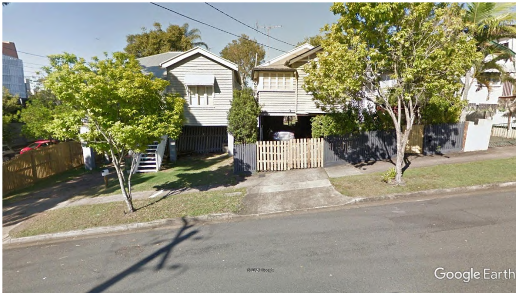
Figure 11 – Typical Properties along Rawnsley Street adjacent to the area where portal works are required
