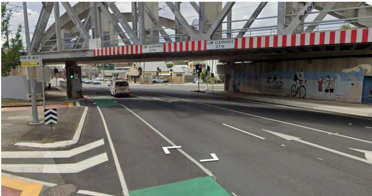
Figure 6-1 Annerley Road Rail Bridge – Low Clearance (3.7m) Point
