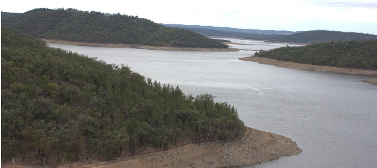
Figure 6-2 Vegetation above the full supply level at Glenlyon Dam
