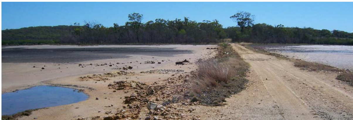
Figure 9.3 - Existing Clarks Road Causeway across Supratidal Saltflats
