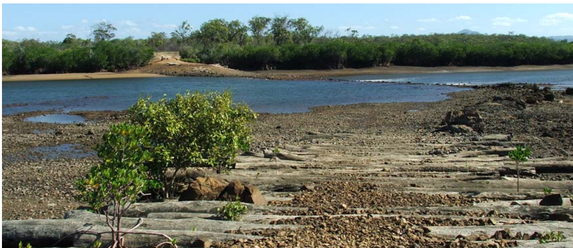
Figure 9.5 – Existing Causeway Across Boyne Creek at Low Tide
