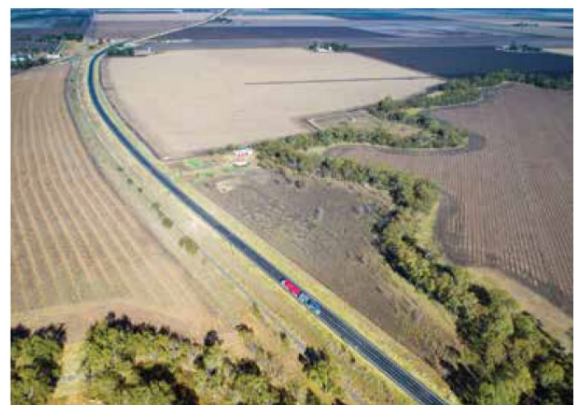
The existing railway line, Gore Highway, Pampas.
