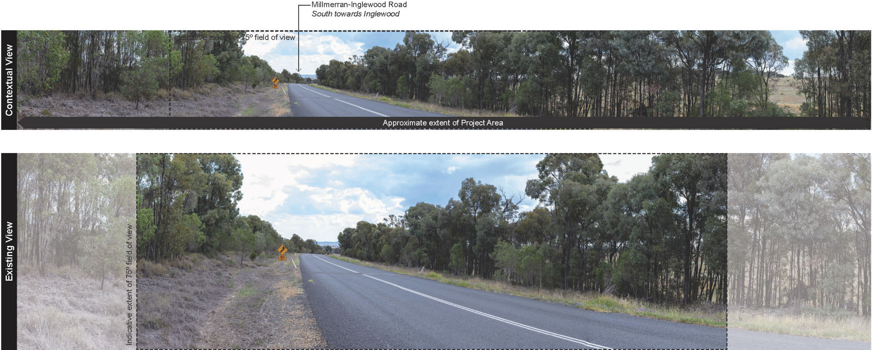
Figure 29: Viewpoint 6: Millmerran-Inglewood Road towards Millmerran-Inglewood Road Rail Bridge #2
