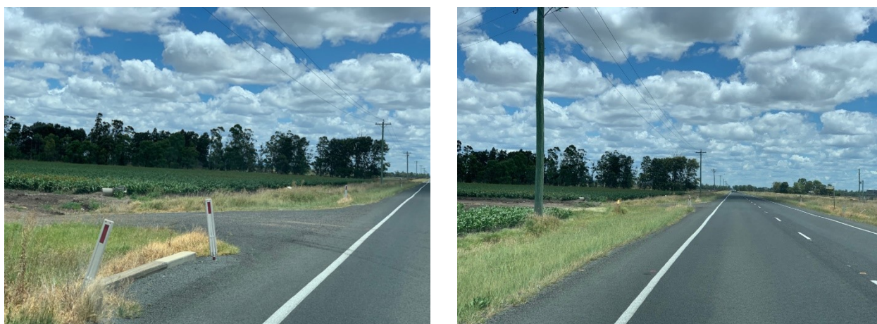
Figure 5.4 Gore Highway/Gilgai Lane site visit photos
