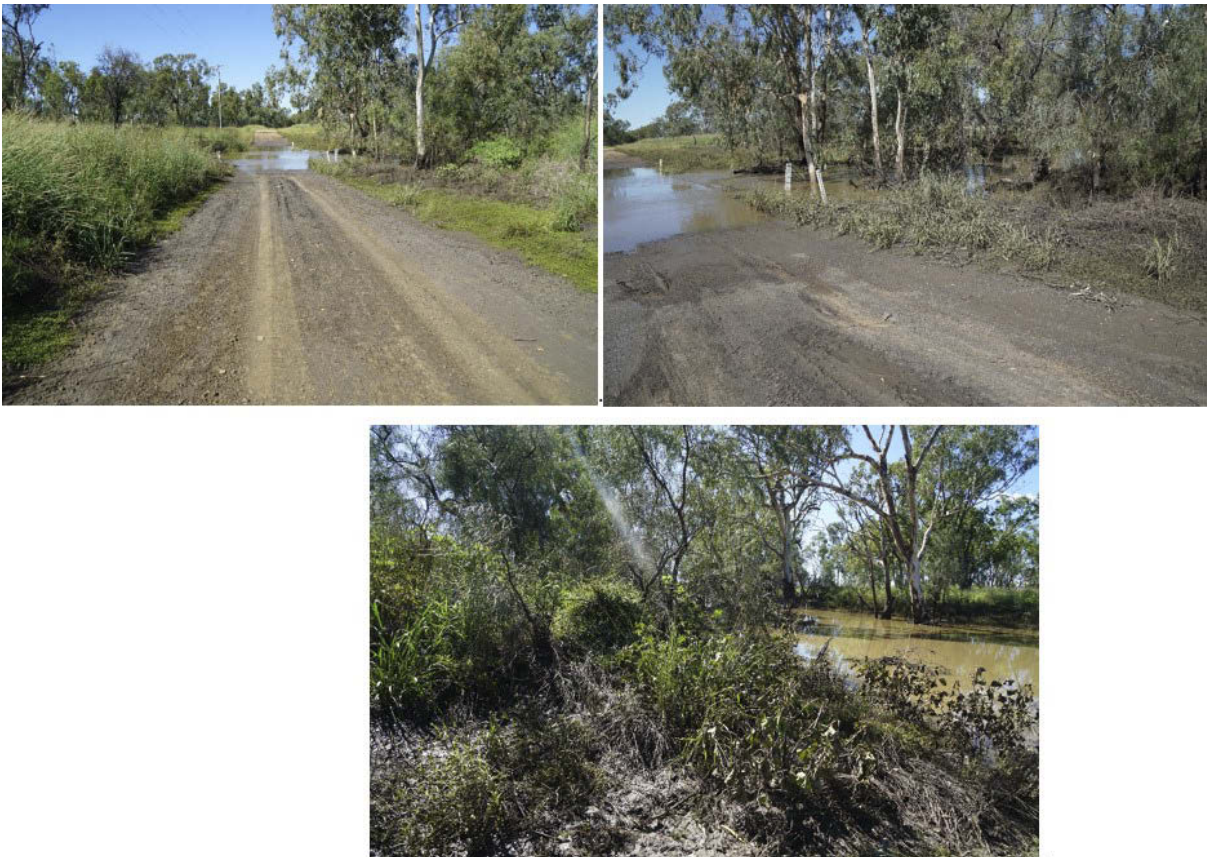
Figure 3.30 Example of 'minor consequence category on Grasstree Creek (field site EP17), approximately 8.7 km upstream of the Project alignment
