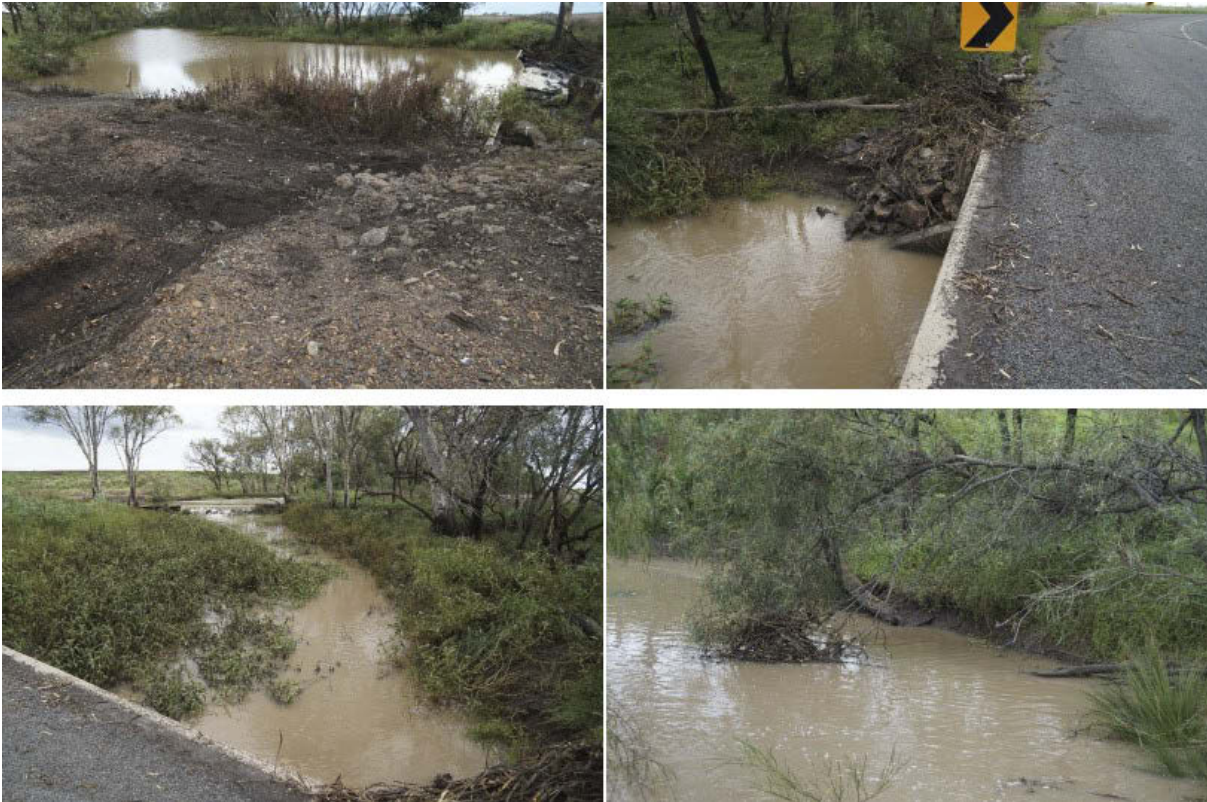
Figure 3.29 Example of 'minor consequence category on the Condamine North Branch (field site 1b), approximately 800 m upstream of the Project alignment
