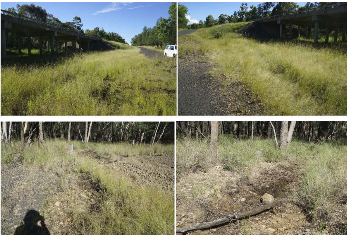
Figure 3.20 Cattle Creek Road bridge site inspection (2/EP34)
