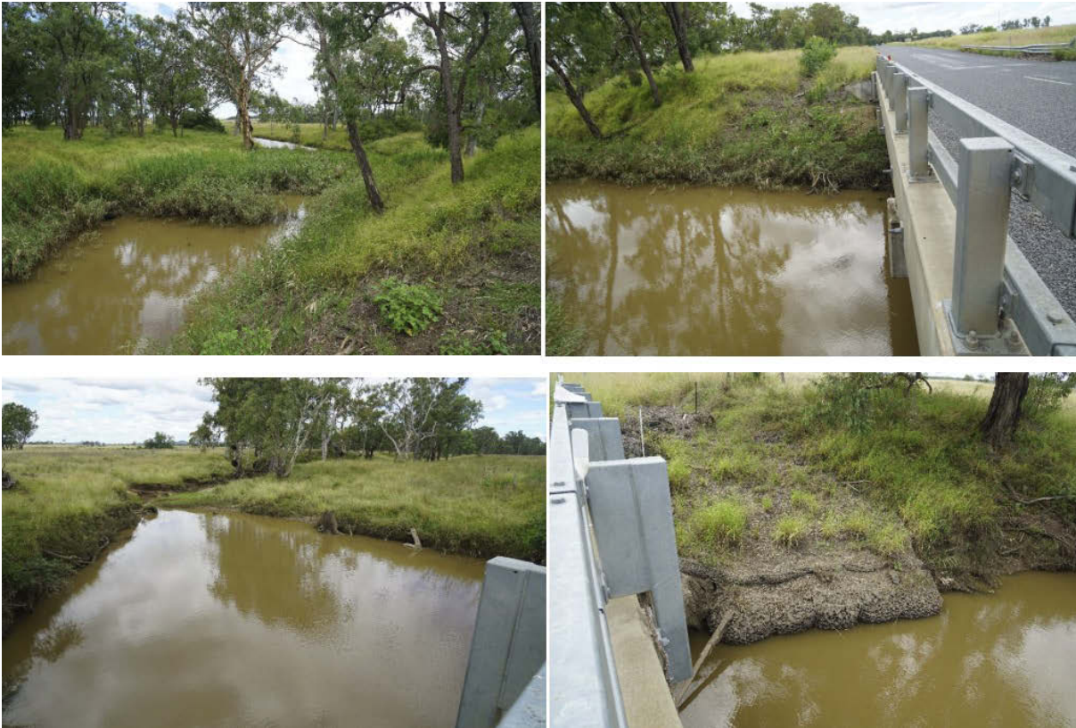
Figure 3.19 Bringalily Road bridge site inspection (EP29)
