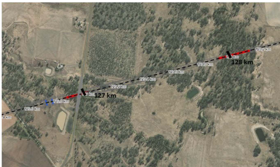
SC 2 floodplain Aerial image
