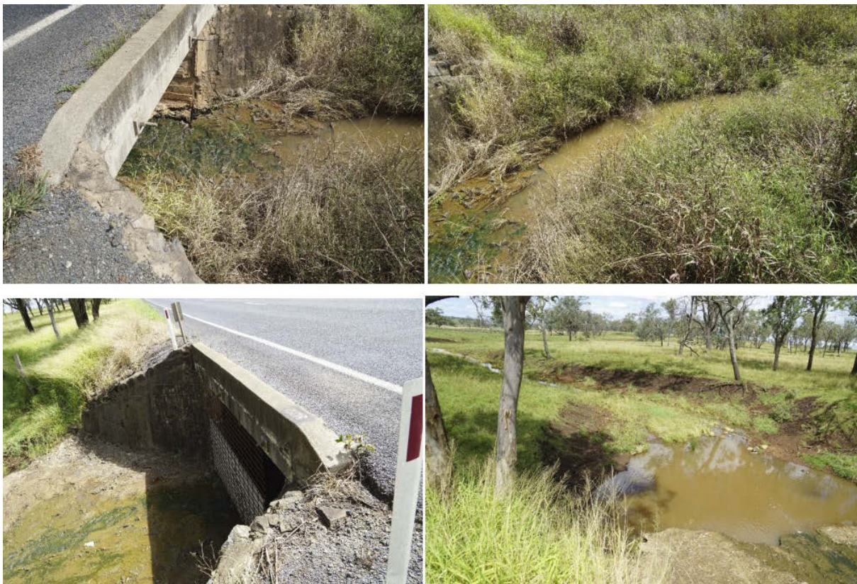
Figure 3.21 Condamine North Branch NC 2 culvert site (EP6) site inspection Cattle creek (2/EP34)
