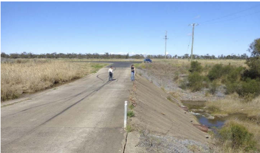
Figure 3.9 Drop structure at Wallingford Road
