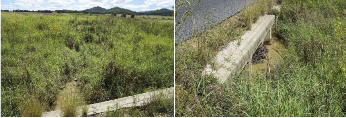
Figure 3.23 Baseline field work site 8, Watercourse SC 5, channel type wash slope/ non-channelised valley floor flow, away from culvert vegetated and stable
