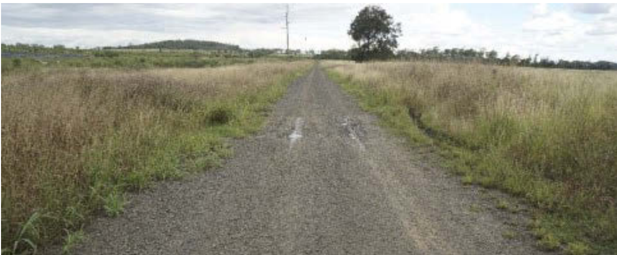
Figure 3.22 Baseline field work site 19, Watercourse (NC 15) flow travels across the road left to right, channel type wash slope/ non-channelised valley floor flow, well vegetated, stable
