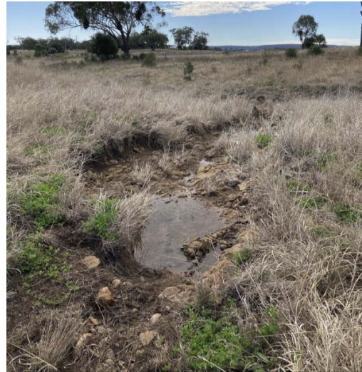
P11 – bank erosion in soil above rock lined channel downstream from culvert (site E3)
