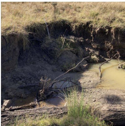
P18 – bank erosion and slumping downstream of road culvert, 1 m white staff for scale (site E4)
