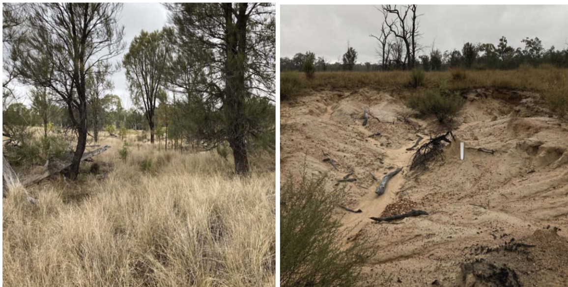
Figure 4 CCs 21 site photos. Left, Photos P1 – looking downstream from proposed culvert location. Right, Photo P6 – gully erosion on side gully at true right of design culvert location.
