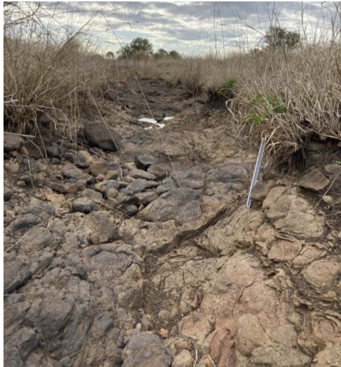
P9 – rock lined channel bed near culvert, 0.25 m white staff for scale
