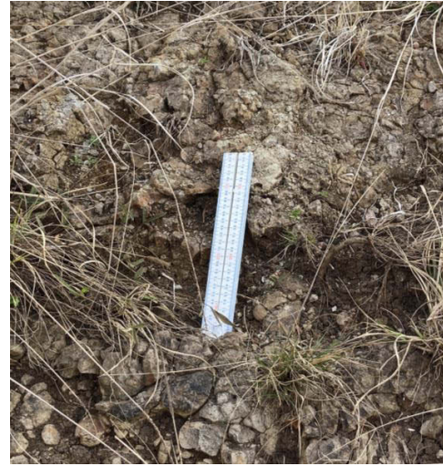
P11 – bank erosion in soil above rock lined channel downstream from culvert (site E3)
