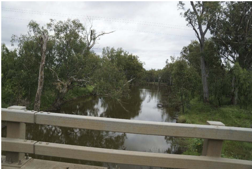
F. 54 EP43 photographs. Downstream northern bridge (top left), upstream northern bridge (top right), downstream southern bridge (bottom left)
