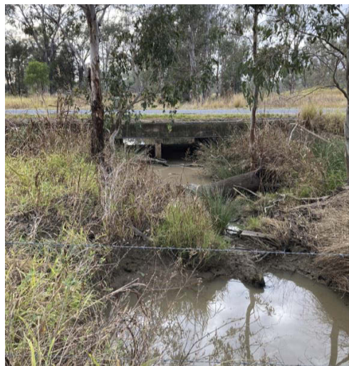
P15 – upstream of road culvert, looking downstream
