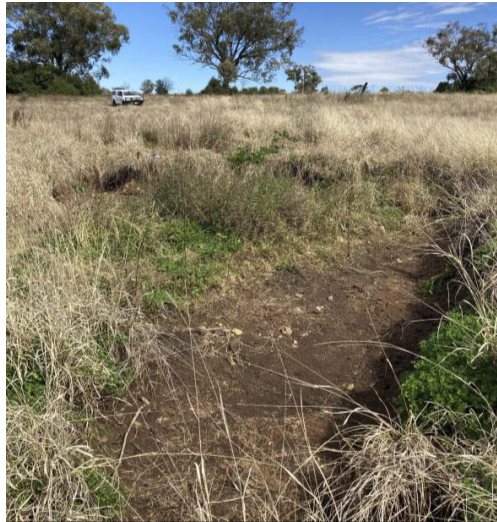
P10 – eroded area in soil downstream from culvert (site E2)
