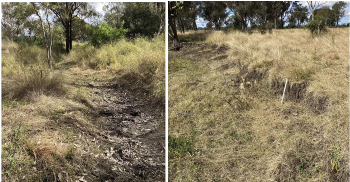
Figure 2 SC 7 site photos. Left, Photos P2 – looking upstream towards proposed culvert location. Right, Photo P9 – minor erosion on true right bank downstream of pond.
