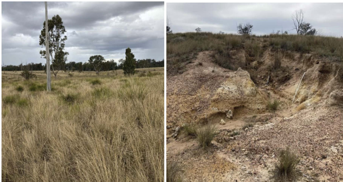
Figure 3 C Ck 16 site photos. Left, Photos P3 – looking downstream towards proposed culvert location. Right, Photo P9 – gulley erosion on side gully downstream of Project alignment, just outside the earthworks area.
