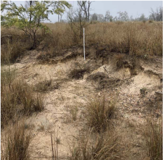
P9 – bank erosion on true right downstream of culvert, white staff for scale 1.0 m (site E14).
