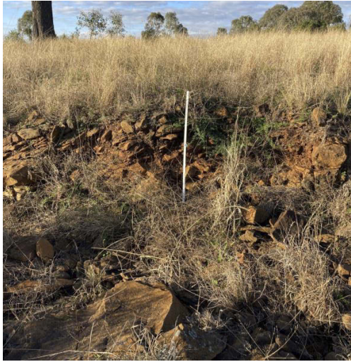
P9 – rock lined channel bed near culvert, 0.25 m white staff for scale
