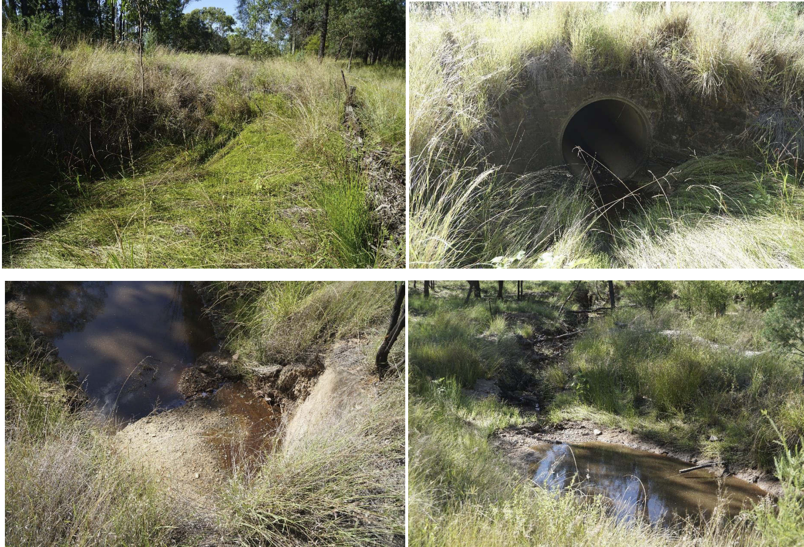
F. 49 EP37 photographs. Upstream (top left), upstream detail (top right), downstream detail 1 (bottom left), downstream detail 2 (bottom right).
