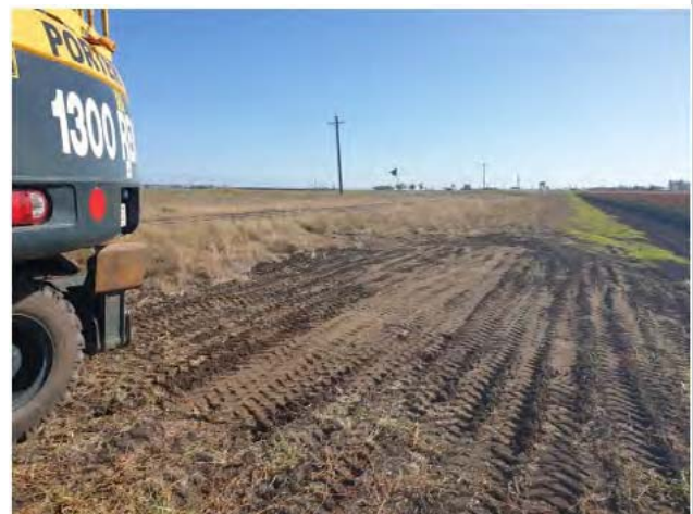
Testpit – Backfilled, Landscape
