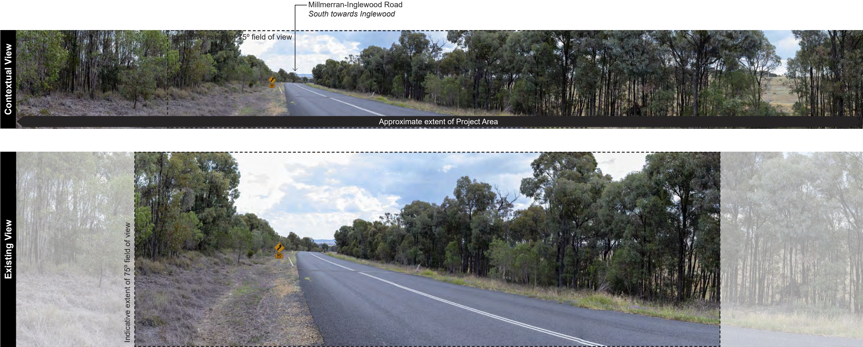
Figure 32: Viewpoint 9: Millmerran-Inglewood Road towards Millmerran-Inglewood Road Rail Bridge #2
