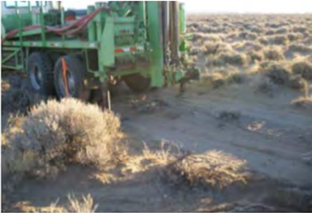
Pre Drilling – truck in position before drilling
