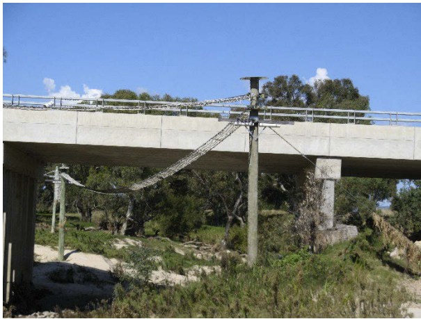
Figure 5.9 Canopy rope bridge under twin bridges on the Hume Highway at Mountain Creek, NSW. Photos Josie Stokes, WSP.
