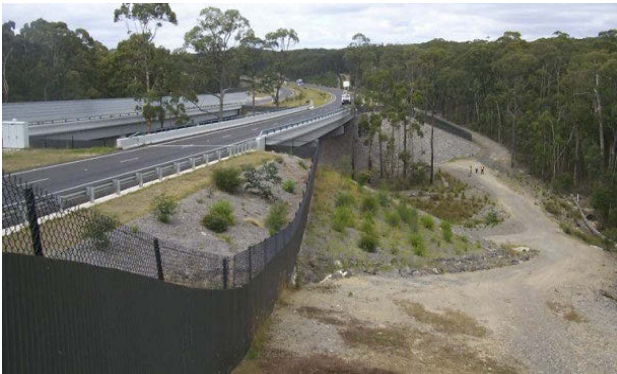
Figure 5.2 The Slaty Creek Bridge on the Calder Freeway in Victoria was designed to be higher and longer than required simply for drainage in order to encourage wildlife movement. In this example, the vegetation has been planted underneath the structures, and tall trees retained between the two carriageways. Photos: Rodney van der Ree
