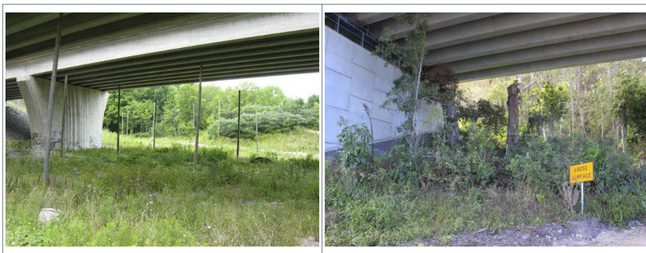
Figure 5.11 (left) Two arrays of artificial glider poles under a road in Ontario, Canada, installed for the northern flying squirrel and (right) retained tree trunks under bridge along Pacific Highway NSW for squirrel gliders, which can also double as a koala refuge pole. Glider poles under bridges should only be used where retained tree trunks are not feasible. Photo at left courtesy of Christine Kelly and right by Rodney van der Ree, WSP.
