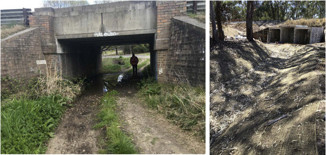
Figure 5.4 Bridge for drainage and vehicle movement under railway at Bowral (left) and drainage culvert at Ettamogah (right) provide incidental movement opportunities for wildlife. Simple improvements such as increasing the width of the bridge and reducing ponding can improve effectiveness for wildlife as well as fulfil its primary function. Photos by Thomas Haffner ARTC.
