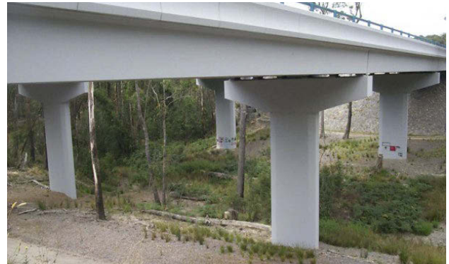
Figure 5.2 The Slaty Creek Bridge on the Calder Freeway in Victoria was designed to be higher and longer than required simply for drainage in order to encourage wildlife movement. In this example, the vegetation has been planted underneath the structures, and tall trees retained between the two carriageways. Photos: Rodney van der Ree
