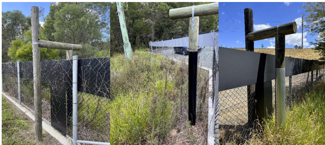
Figure 5.18 ‘n’-shaped koala escape pole (two-way escape pole), shown from (left) the road- or railway-side of the fence and (middle and right) the habitat side of the fence. The pole on the habitat side of the fence includes plastic or sheet metal wrapping that prevents koalas from climbing into the transport reserve. Sheet metal is also attached to the fence at the pole to prevent climbing up the fence and then the pole above the wrapping. Escape poles can also terminate at the top of the wrapping, requiring koalas to jump down. ‘Two-way’ escape poles do not have plastic or sheet metal, allowing fauna to use the structure in either direction. Photos Rodney van der Ree.
