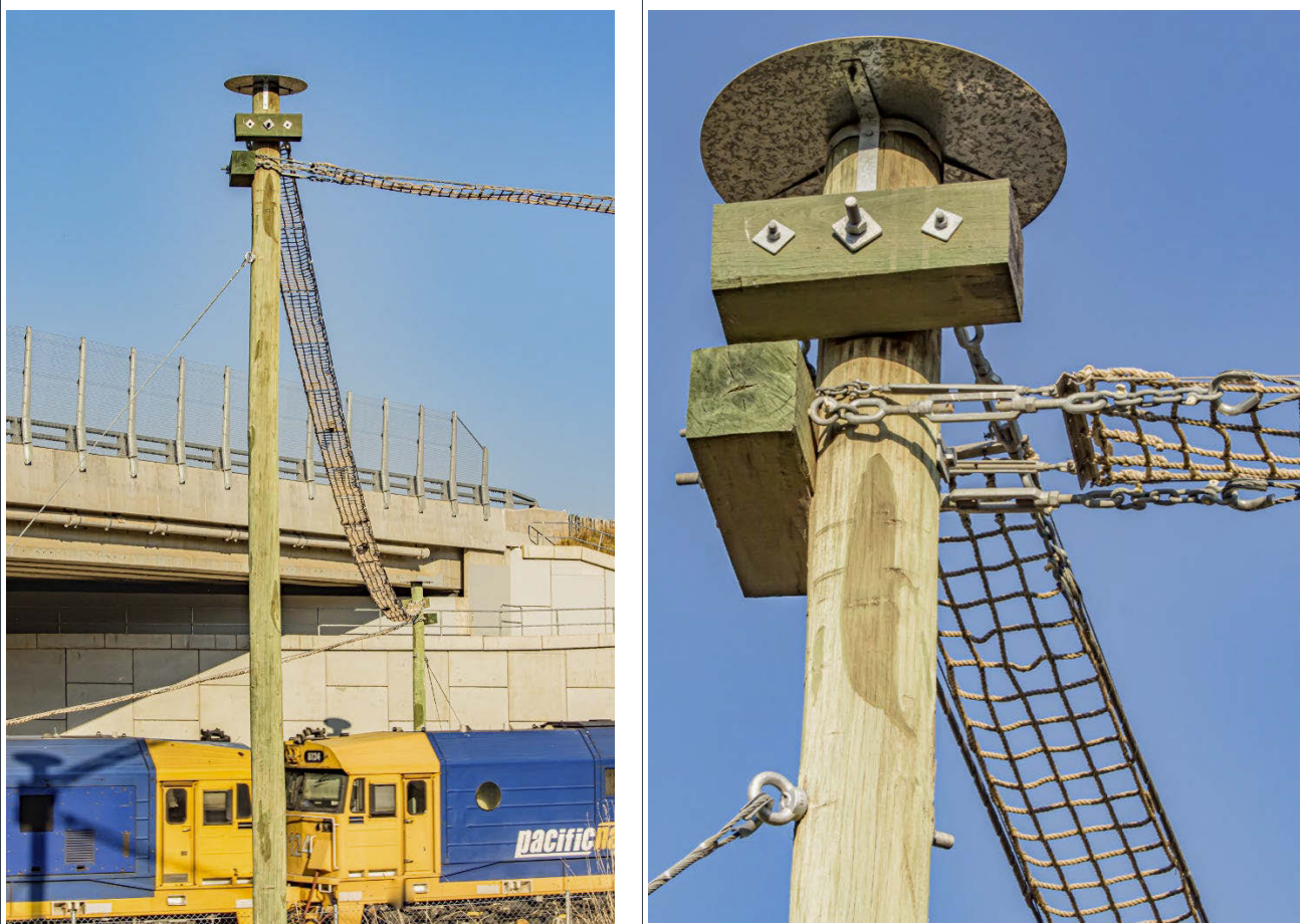
Figure 5.8 Canopy rope bridge across the railway and under the Olympic Highway at Kapooka, NSW, showing the flat rope ladder attached to two steel cables, as well as the predator shield and attachment detail. Photos by Allan Richardson, WSP.
