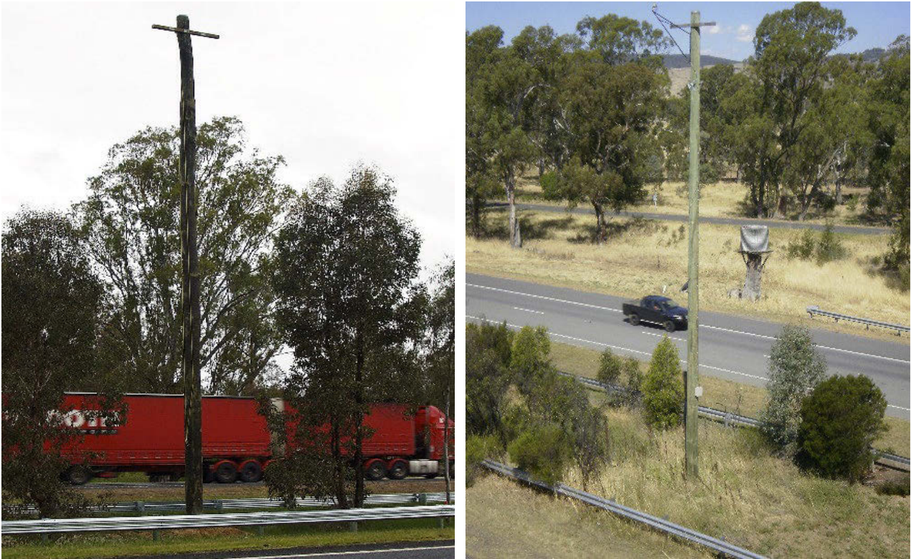
Figure 5.10 Glider poles installed in the centre median of the Hume Freeway, Victoria. Note that the cross-arm should be perpendicular to the road or railway and point towards the opposite side of the infrastructure. Photos by Rodney van der Ree, WSP.
