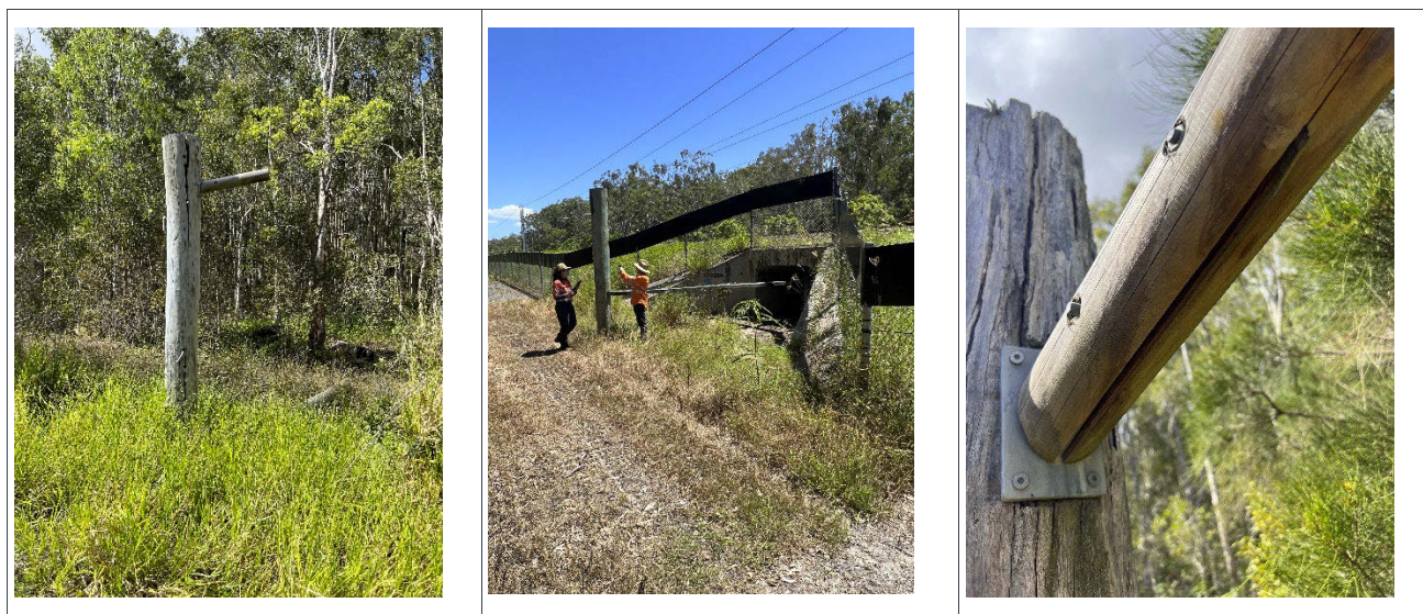
Figure 5.12 Koala refuge pole constructed from recycled telephone pole (left), treated pine at end of koala rail (middle) or salvaged tree trunks. Photo on right shows one method to attach the fork to provide a resting spot for koalas. Photos: Rodney van der Ree.
