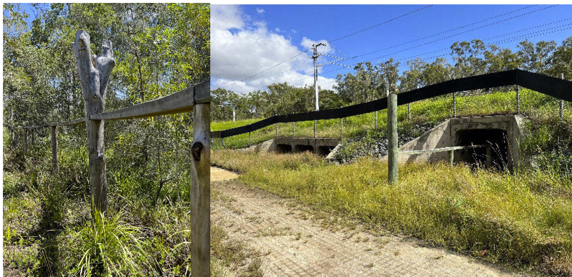
Figure 5.13 Koala rails installed in approach areas to culverts and bridge underpasses. Note the use of salvaged tree trunks as part of the railing (left) also providing a refuge function. In this installation, animals must climb up and over the trunk, potentially reducing ease of use. Overgrown vegetation may also reduce function. Photos: Rodney van der Ree.
