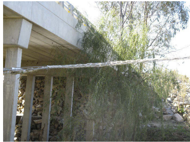
Figure 5.9 Canopy rope bridge under twin bridges on the Hume Highway at Mountain Creek, NSW. Photos Josie Stokes, WSP.
