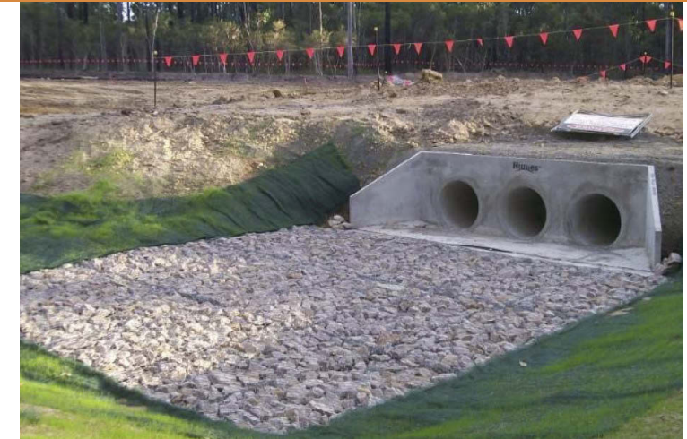
Rock revetment mattress—Culvert outlet application (Global Synthetics, 2020)
