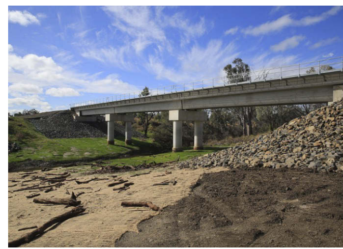
Finished Croppa Creek Bridge with rehabilitated riverbank (ARTC, 2022)
