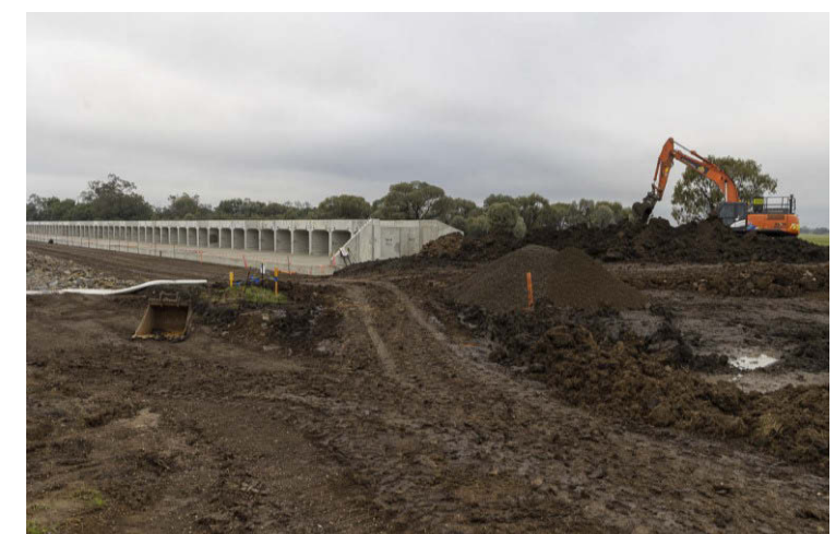
Backfilling the culverts as part of the formation works south of Moree (ARTC, 2022)
