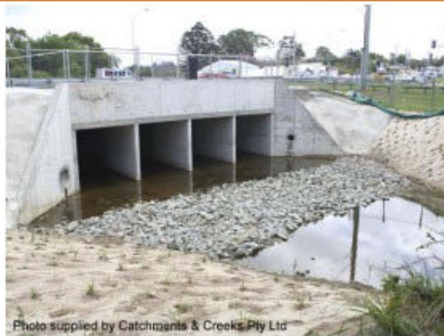
Erosion and scour rock protection at culvert outlets (Catchments and Creeks Pty Ltd)
