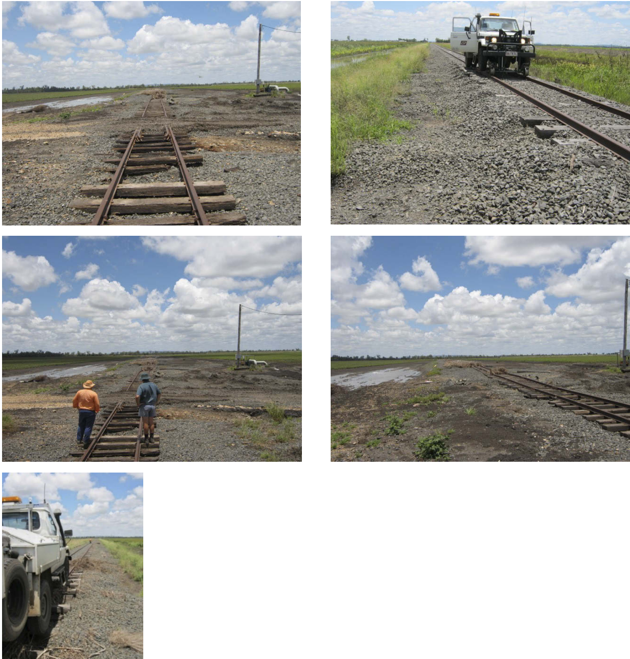
Figure 7.57 Condamine River floodplain—Evidence of historical debris deposition and scour provided by Queensland Rail (actual flood event unknown)
