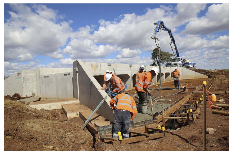
Concrete pour as part of the drainage construction ('apron') (ARTC, 2022)
