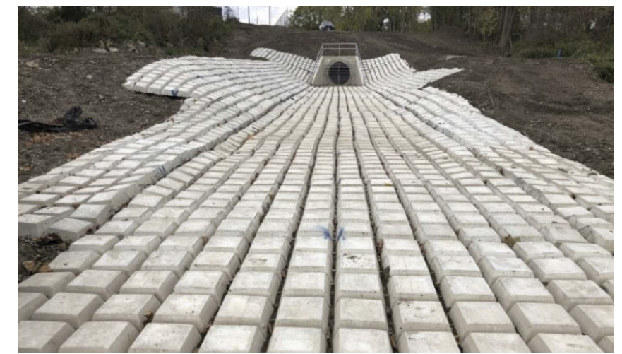
Flexible concrete mattresses (IECS, 2023)
