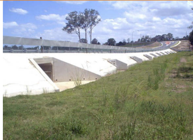
Spaced culvert cells to spread flow (ARR 2019)
