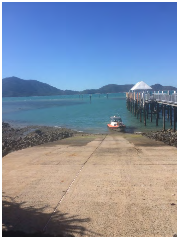
Photo 4: Slipway and jetty at near low tide level
