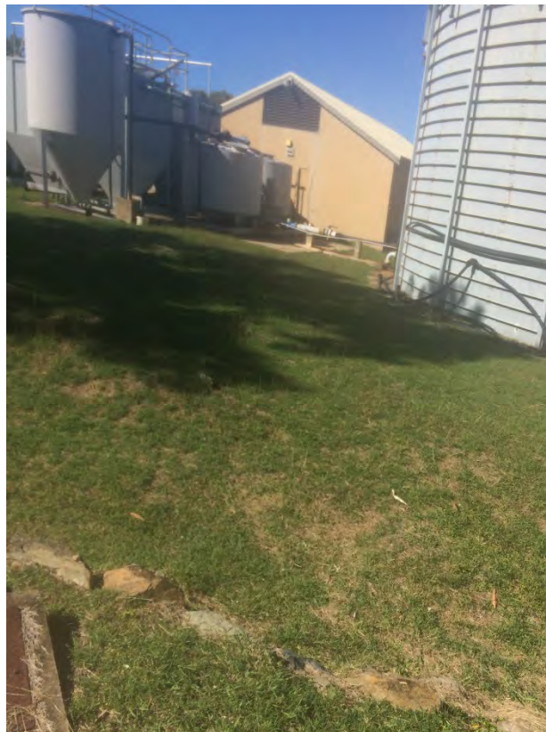
Photo 2: Tank and workshop area
