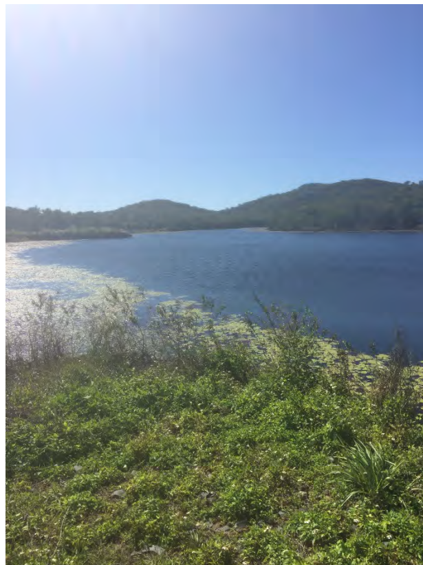
Photo 8: Main dam pond looking north
