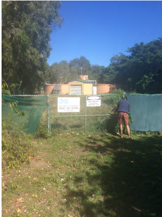
Photo 3: Old sewage treatment plant
