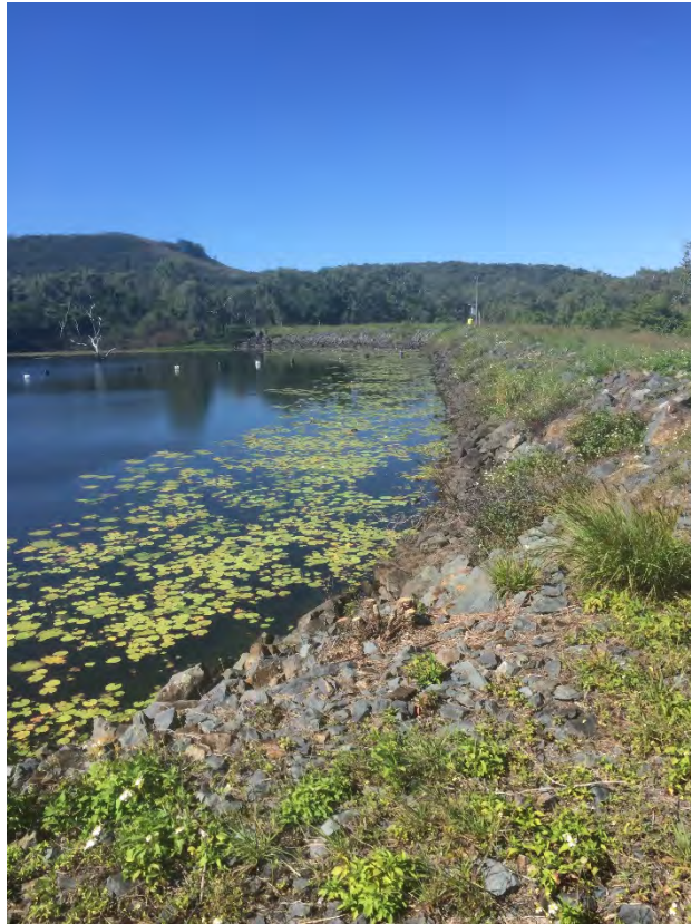
Photo 9: Dam upstream well
