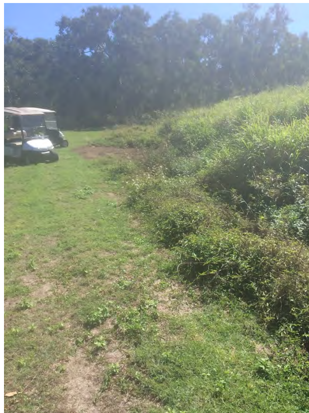
Photo 16: Downstream wall of blackwater dam
