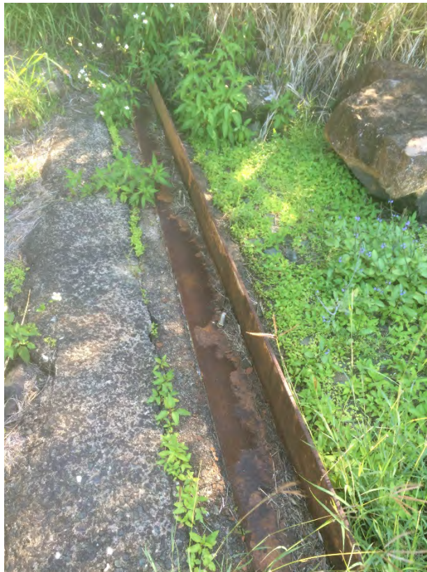
Photo 10: Spill wall lip on dam
