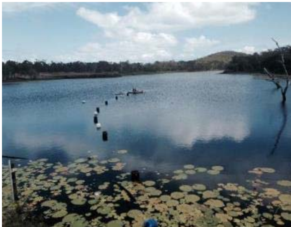
Figure 3-8. Gap Creek Dam.
