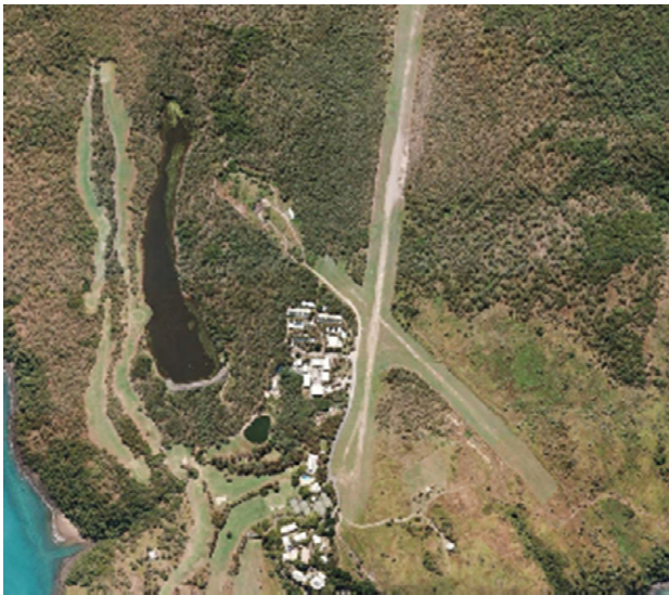
Figure 4-11. Existing aerial photograph of Tourist Villa Precincts.
