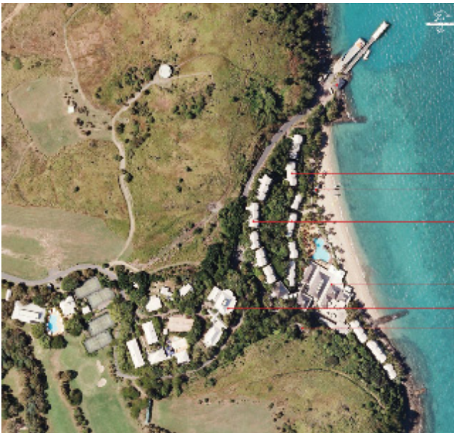
Figure 4-2. Existing aerial photograph of Beach Resort locality.
