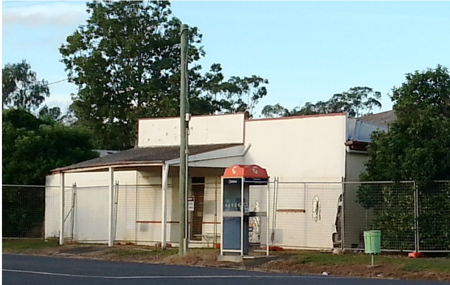
Photo 5 - Derelict former Acland store prior to demolition.
