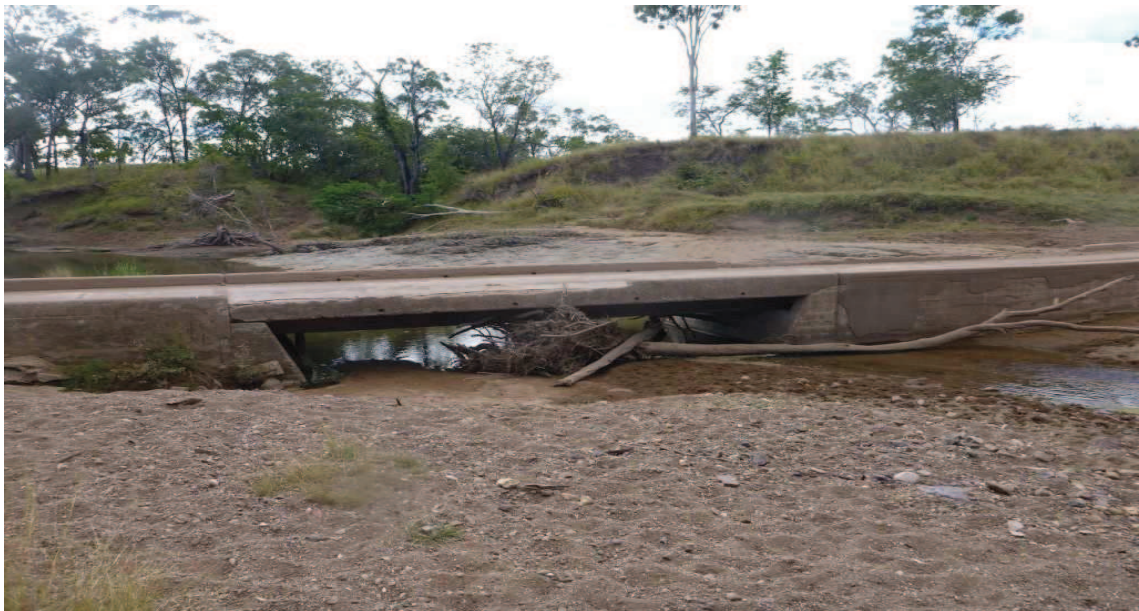
Photograph 3.6 – Strathmore Creek at Strathmore Road
