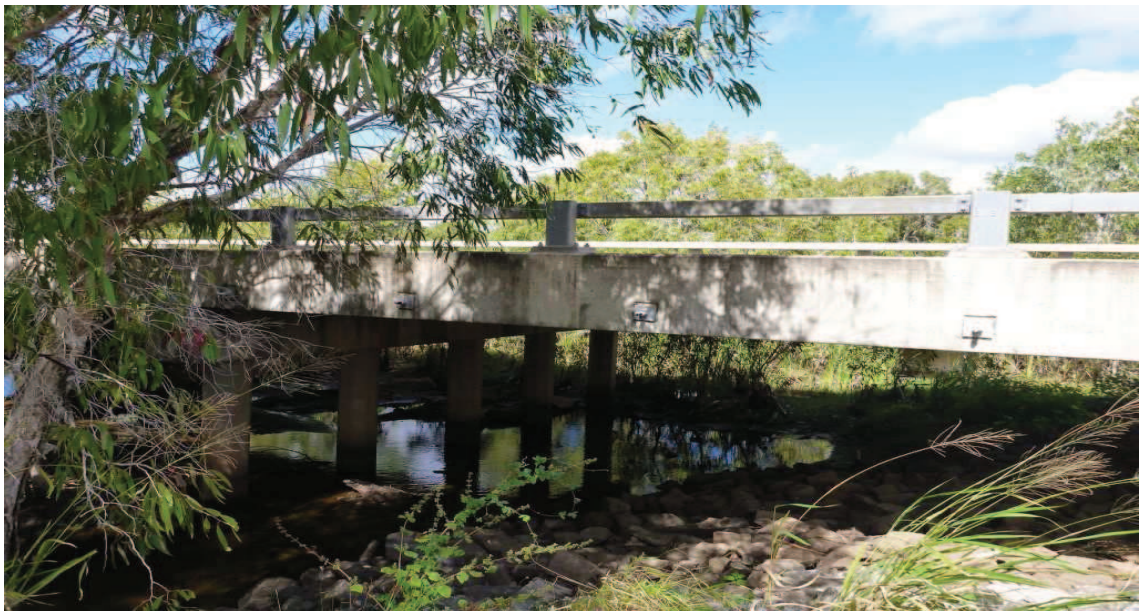
Photograph 3.3 – Salt Water Creek at Bruce Highway
