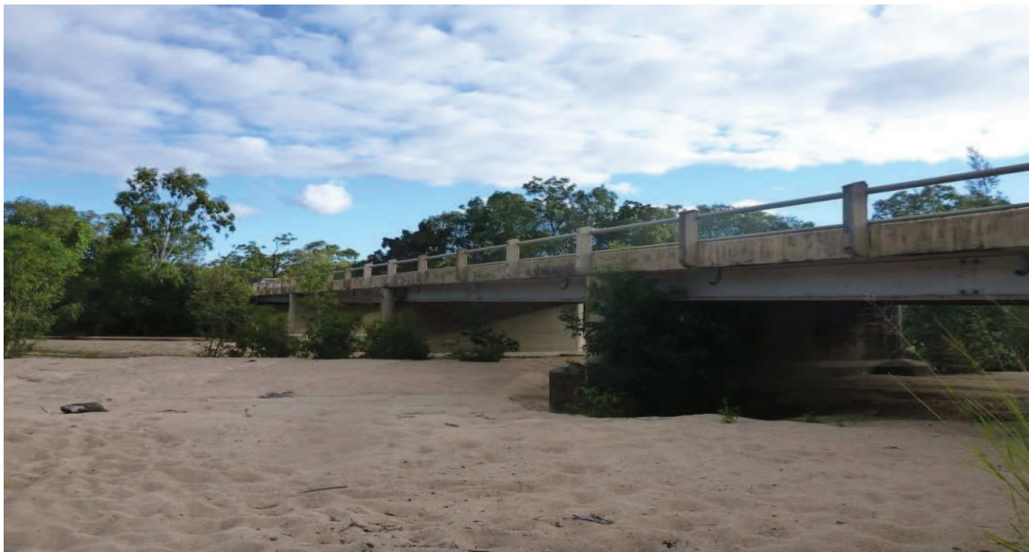
Photograph 3.5 –Bogie River at Bowen Developmental Road
