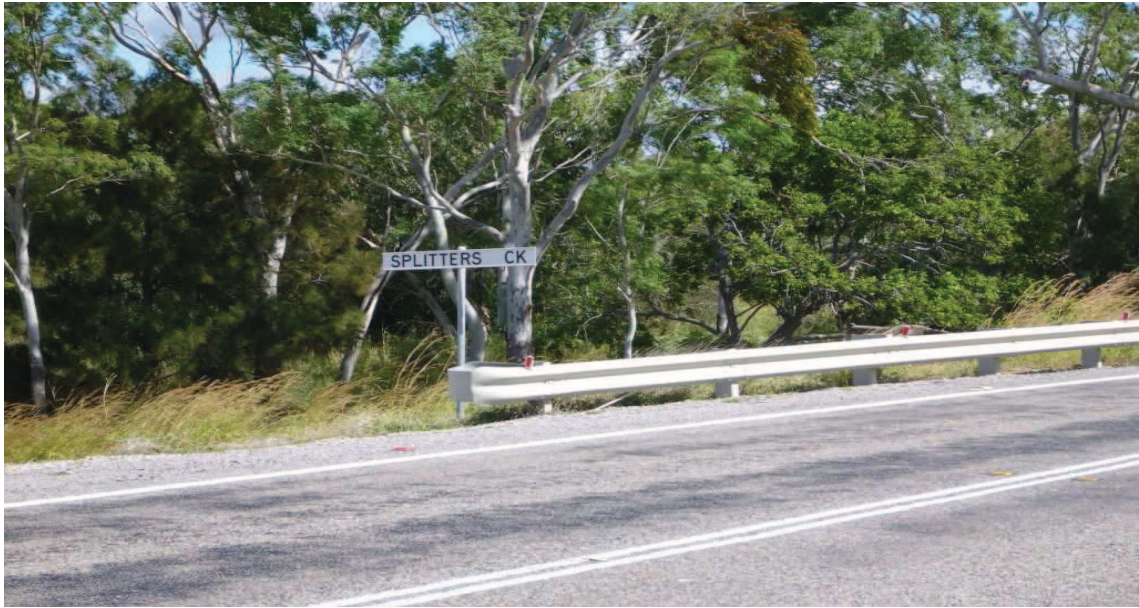
Photograph 3.2 – Splitters Creek at Bruce Highway
