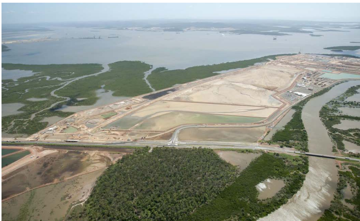
Figure 5.2 Wiggins Island Reclamation Area B (April 2013)
