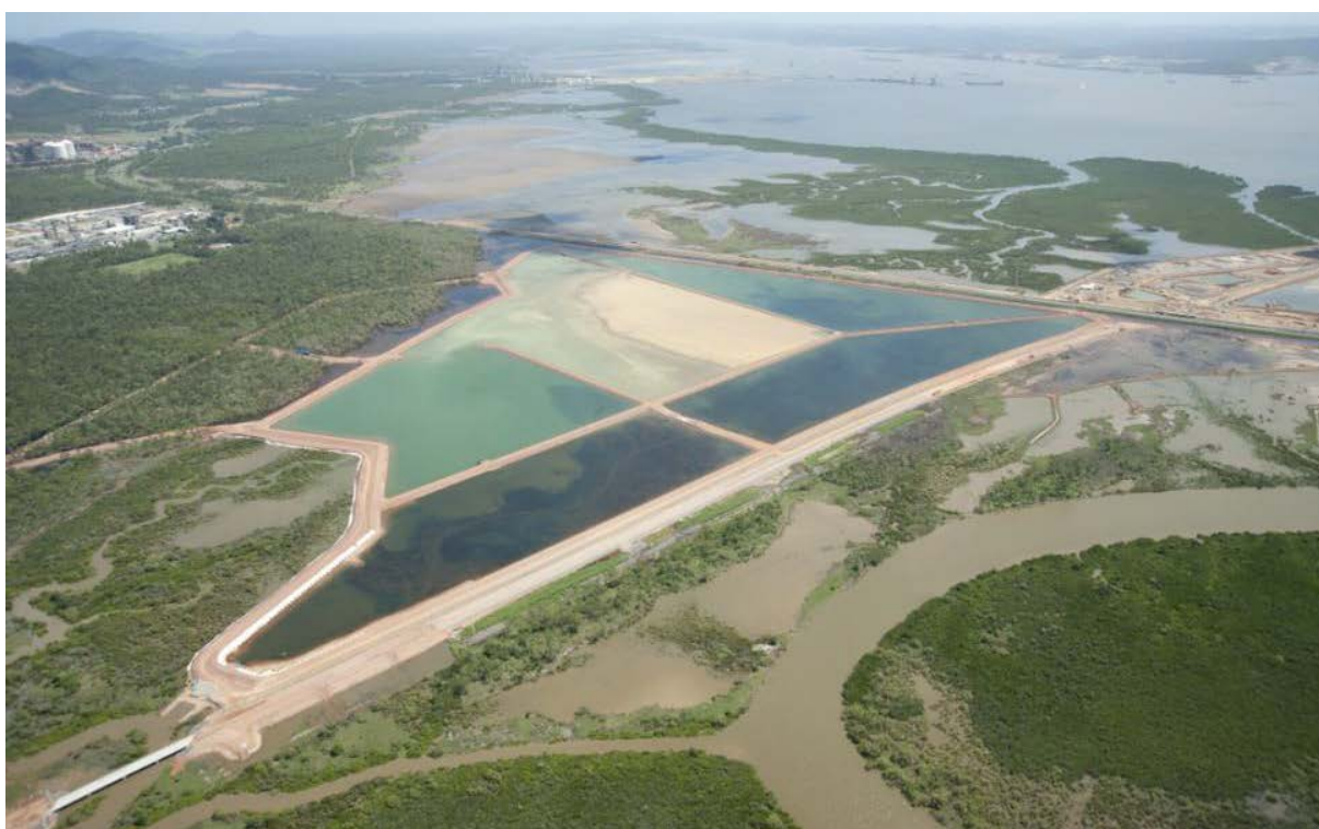
Figure 5.3 Wiggins Island Reclamation Area C (April 2013)
