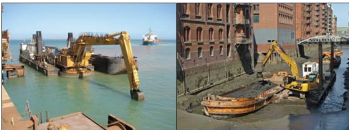
Figure 4.3 Examples of back hoe (left) and grab dredgers (right)
