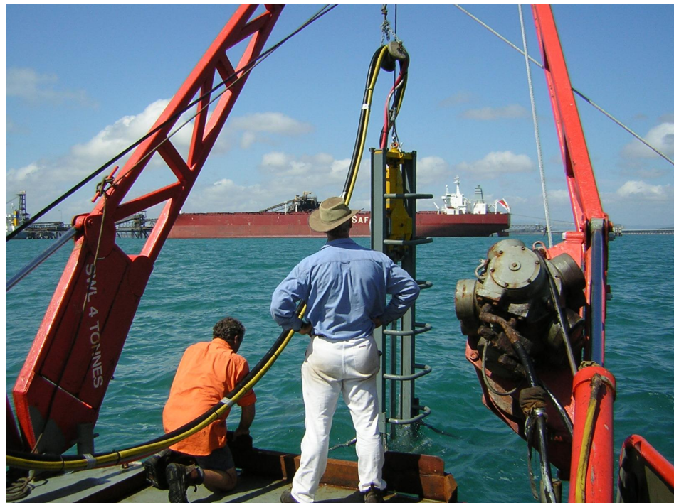
Figure 3 Vacuum Vibrocorer
