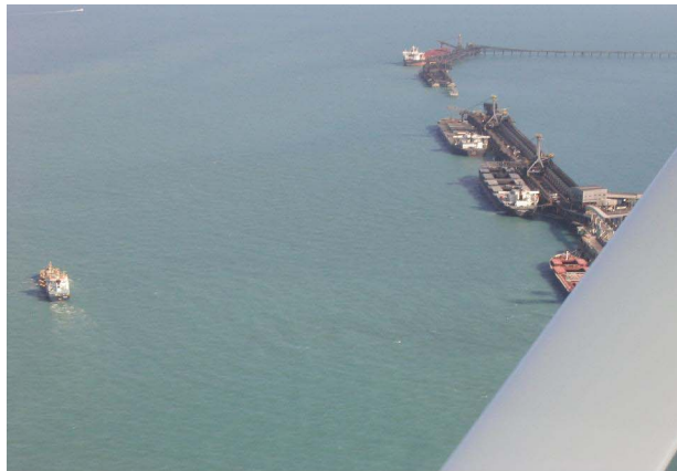
a. Photo 1: 3:30 pm – The dredger was operating along the DBCT
