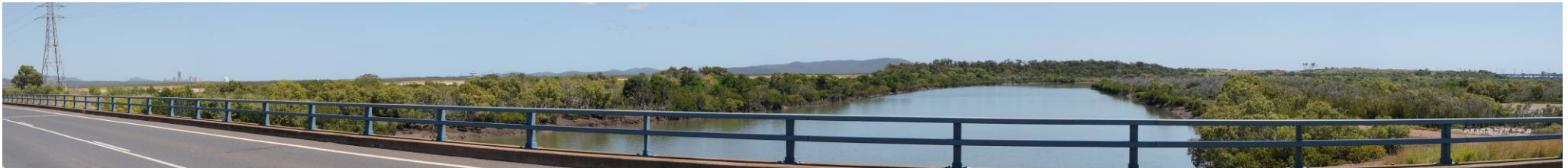
Photograph 8.13 View looking north from Port Curtis Way at the bridge over the Calliope River Anabran.
