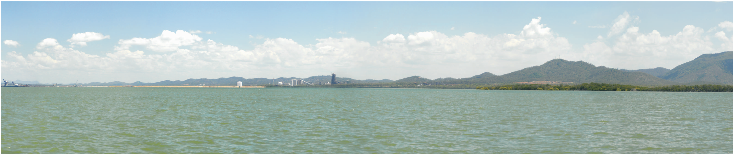
VIEW LOOKING SOUTHWEST TOWARDS TARGINIE, AT APPROX 1KM FROM THE PROPOSED LOCATION OF THE CURTIS ISLAND BRIDGE
