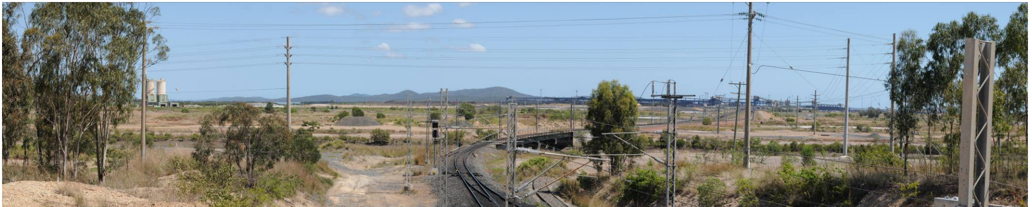
Photograph 8.12 View looking north from Port Curtis Way, approx 3km to the west of Gladstone City centre.
