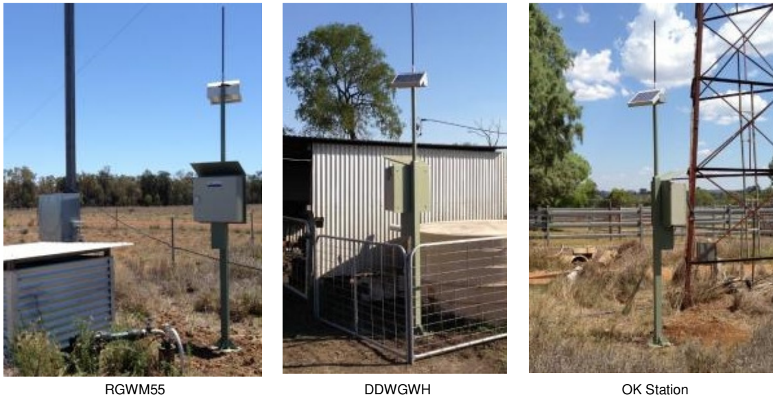
Figure 7-3: Private Bores Equipped with Telemetry
