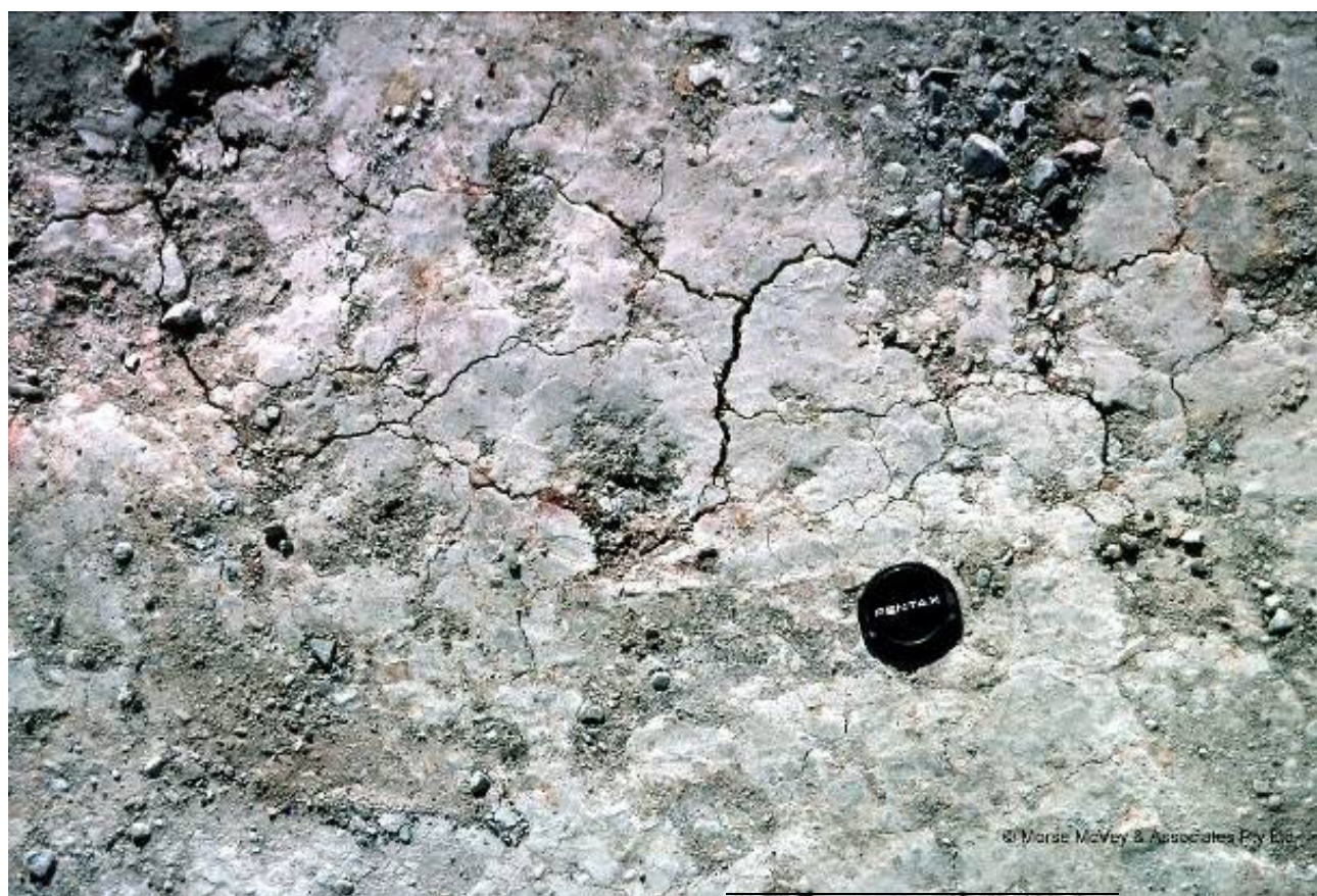
Photograph A3-1 Compacted and smooth surface condition on a construction site.
