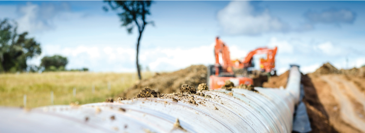
Santos GLNG's gas transmission pipeline under construction near Banana, Queensland, in mid-2013.
