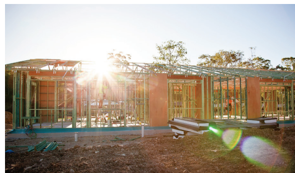
Santos GLNG housing under construction in Gladstone.
