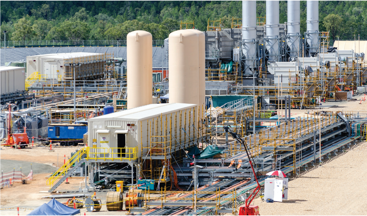
Plate 3–2 Construction of a co-located water treatment and gas compression facility at Fairview
