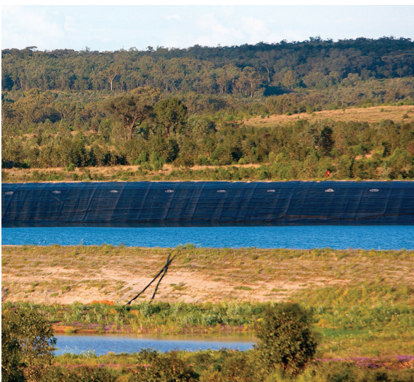
A water storage facility at Coxon Creek, Wallumbilla North, Queensland.
