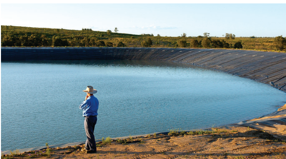
Water storage at Coxon Creek, Wallumbilla North, Queensland.
