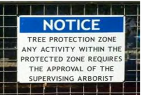
Image 1 – Temporary Metal Exclusions Fencing and Exclusion Zone Signage (Source Arbor Australis)
