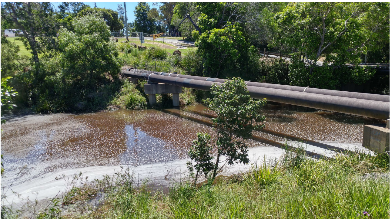
Figure 6: High flow in Six Mile Creek immediately downstream of Six Mile Creek Dam
