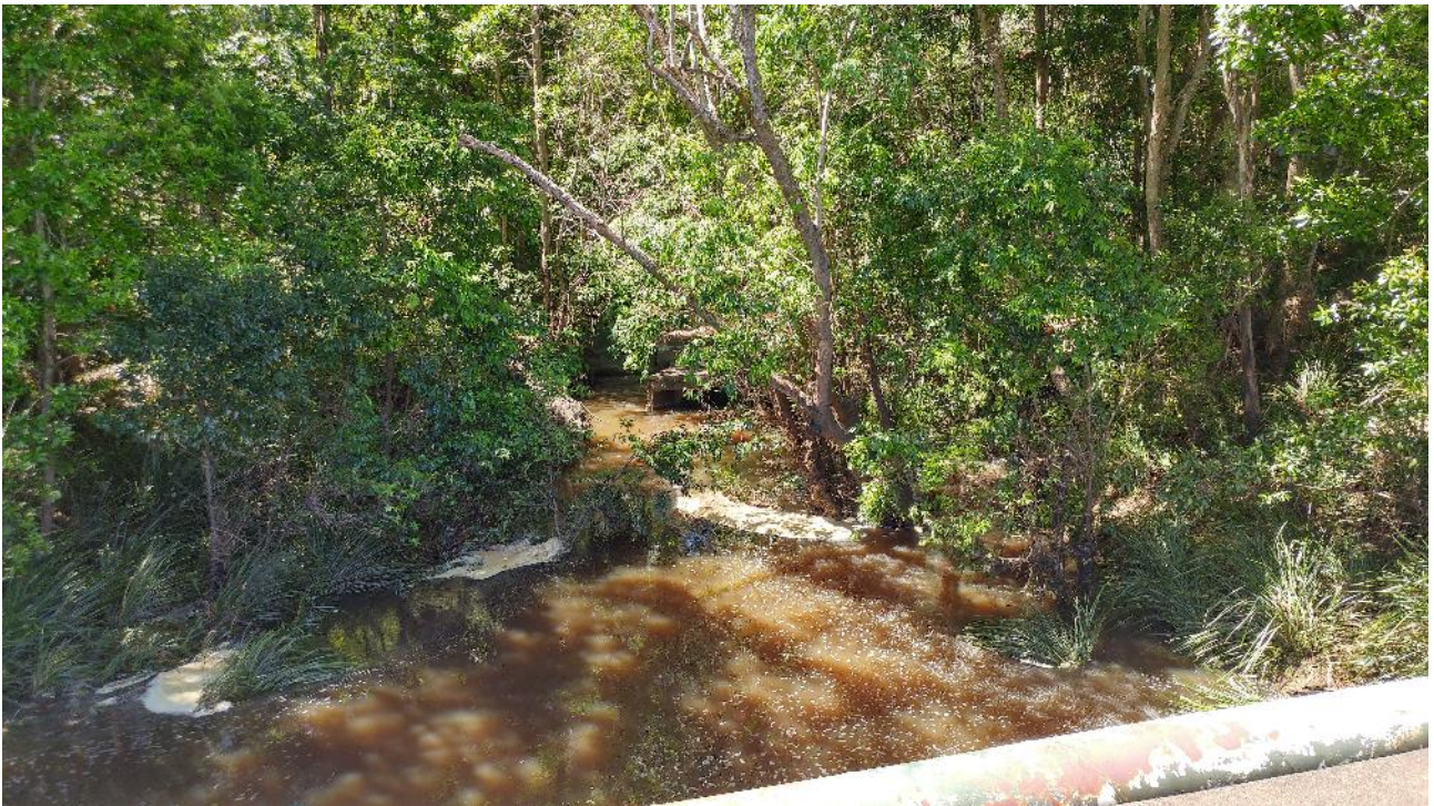
Figure 5: High flow in Six Mile Creek downstream of Six Mile Creek Dam
