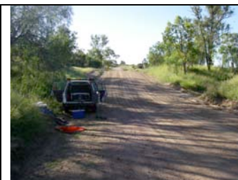
The road crossing did not have culverts
