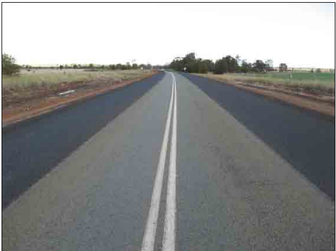
Photo 3-5: Leichhardt Highway — newly ressealed shoulders
