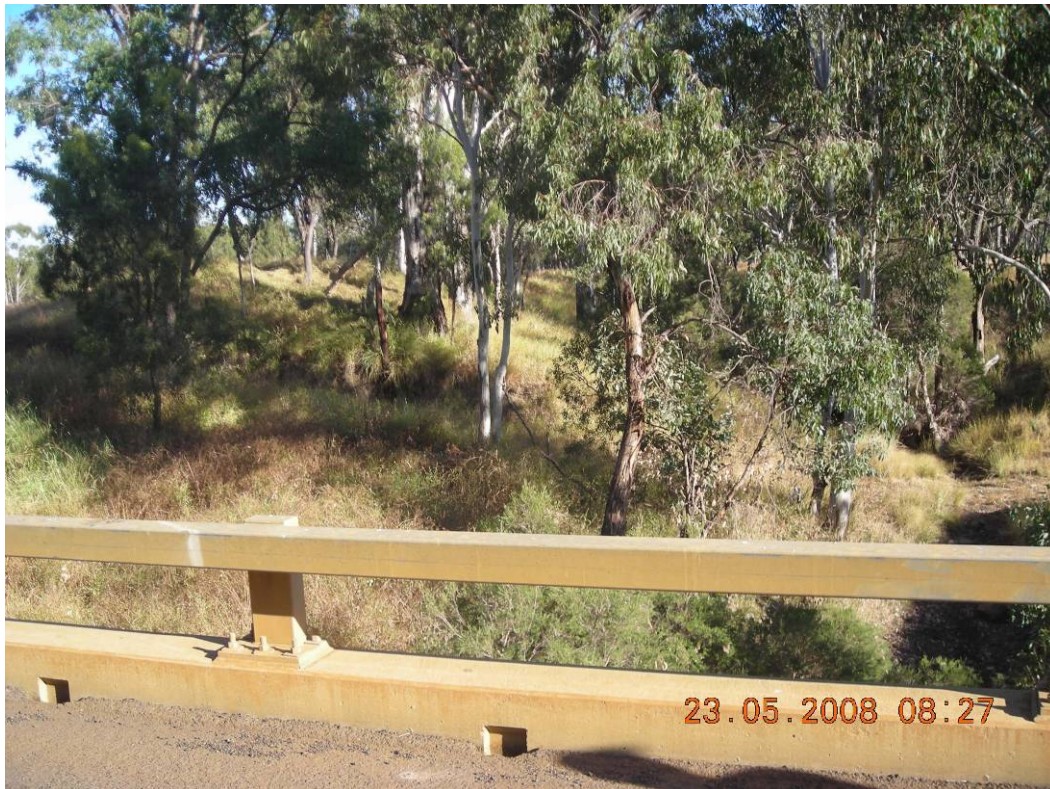
Plate Pipeline 23. Left bank of Cockatoo Creek looking downstream showing nature of bridge and bridge railings (56J 213950E 7157430N)
