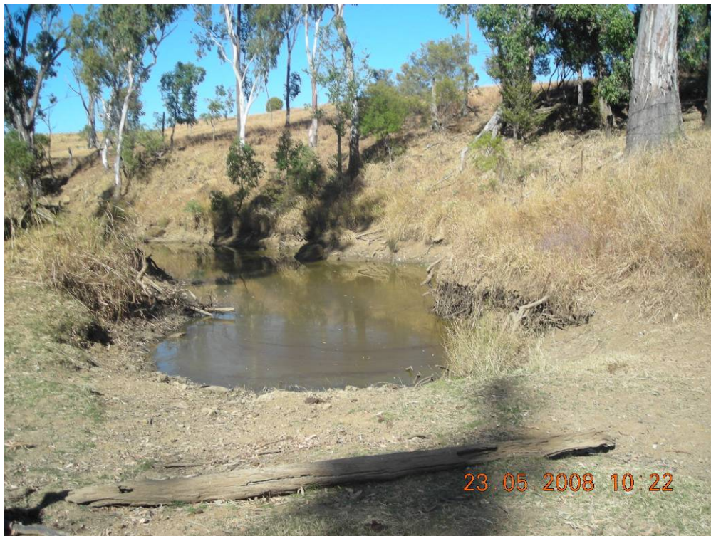
Plate Pipeline 49. Bungaban Creek just upstream of causeway showing rock at water's edge in shadow and upstream and elevated left bank (56J 206870E 7138470N)
