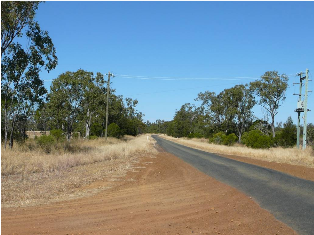
Plate Pipeline 61. Cleared paddock to east with poplar box, false sandalwood and occasional belah in road reserve in Segment 20 with power pole east of road and transformer poles to west (55J 798430E 7120750N)
