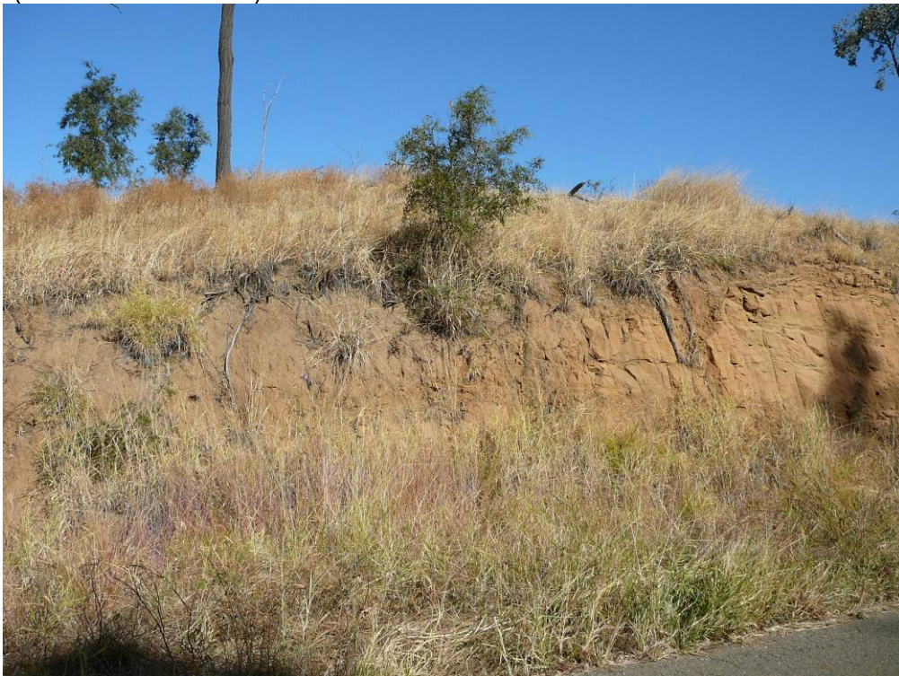
Plate Pipeline 52. Cutting on left bank on southern side of Bungaban Creek showing sandstone sloping down from right to left and overlain by alluvium (56J 206870E 7138470N)
