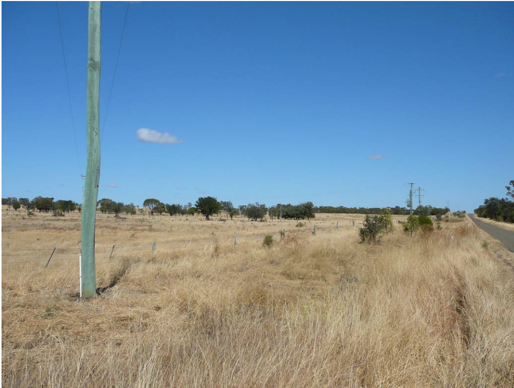
Plate Pipeline 67. Power lines crossing road reserve in Segment 22 with line poles and transformer pole in road reserve (55J 797820E 7117360N)
