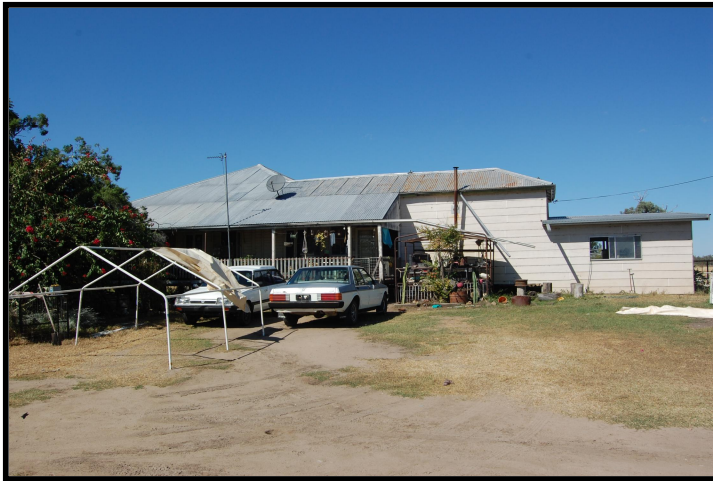
Figure 2-3 North side of the Booral house showing hardiplank clad extension and aluminium window. Photograph by BCA 2008.
