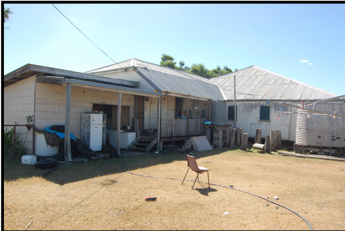
Figure 2-4 West side of the Booral house showing some of the original weatherboard cladding, sash window, exposed beam wall of the core and ant capped stump. Photograph by BCA 2008.
