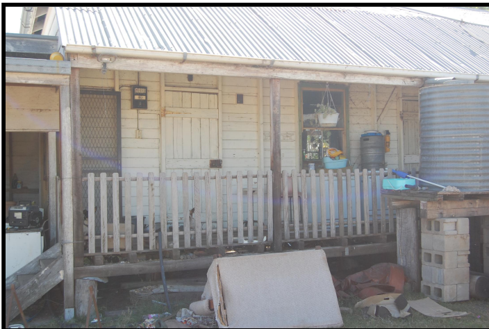
Figure 2-5 Closer view of some of the original elements extant on the west side of the Booral house. Photograph by BCA 2008.
