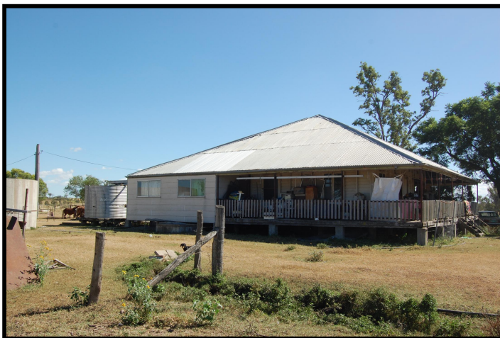
Figure 2-2 South side of the Booral house showing modifications: hardiplank cladding and aluminium windows. Photograph by BCA 2008.
