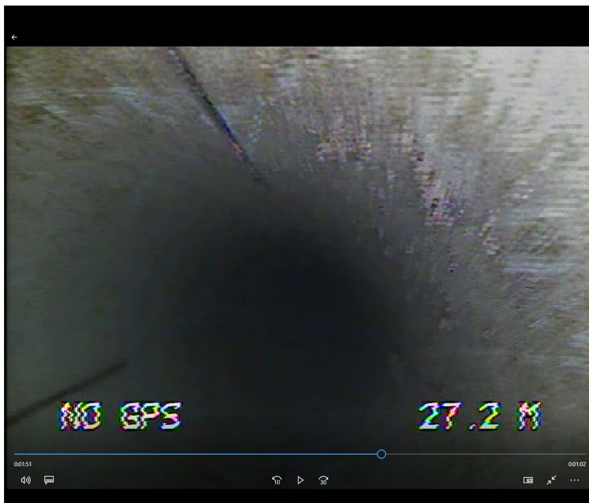
Photograph 3 (slotted casing, Bore 11A) refer in APPENDIX E
